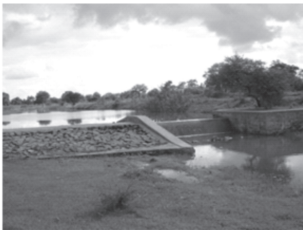
Fig. 2. Boulder check dam at the upper reaches (Kurudih village)
