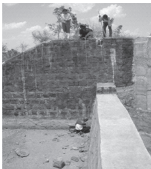
Fig. 5. Measurement of dimensions of recharge structures in the study area
