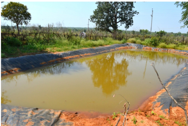
OFR with capacity of 600m 3
