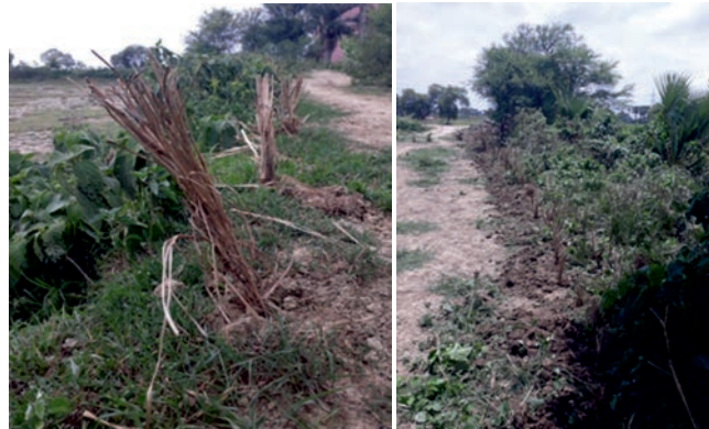
Figure: Biological treatment of the pond embankment for strengthening and creating recreational and aesthetic value.
