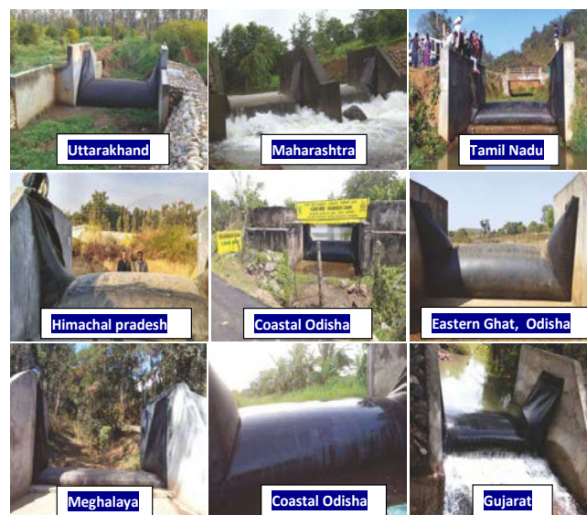
ICAR Flexi-check dams installed in different agro-ecological regions of the country
